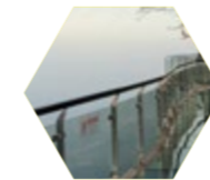
阳台护栏 Balcony railing glass
